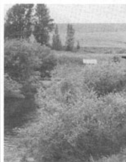
This upper section of the Marysville Canal would be eliminated by the installation of a pipeline system.
